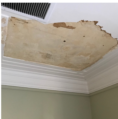
Northeast corner of ceiling
